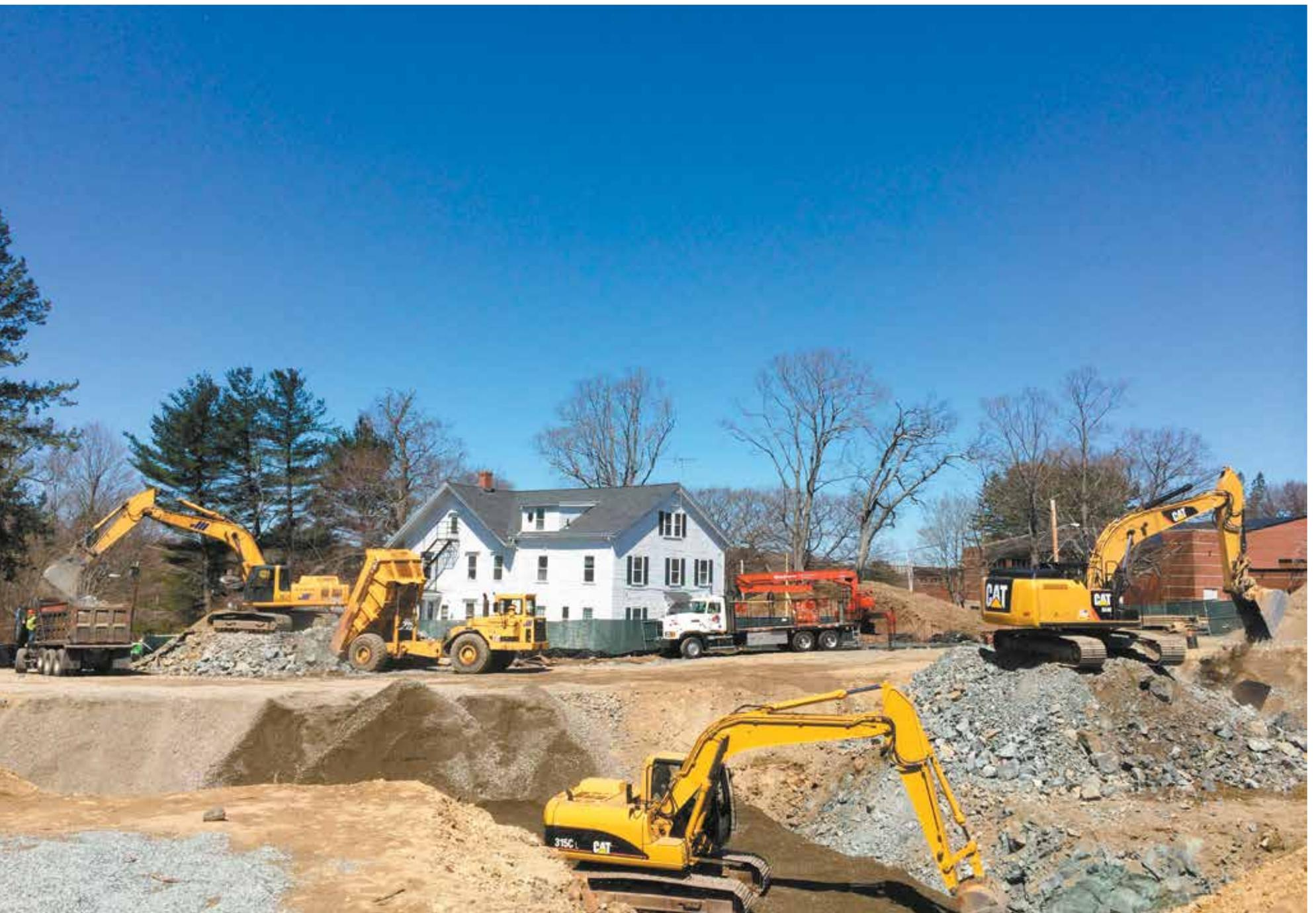
CAT 315C, 324E, 330C Excavators and a D25C Off-Road Truck are used to clear out rock blasted by J Masterson, the site contractor for new science building.
