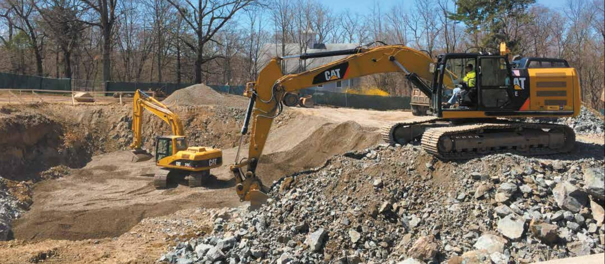
Glacial till and weathered bedrock is removed by Cat excavator which will be followed by placement of engineered base material to support new building footings and walls.
