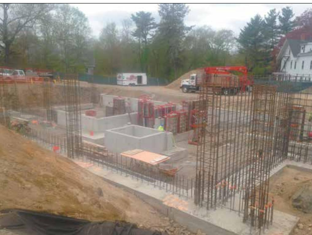
Heavy rebars await placement of forms and ready mix pour for high walls around basement.
