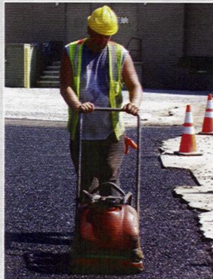
Victor Miraud from Aggregate Industries compacts the edge.
