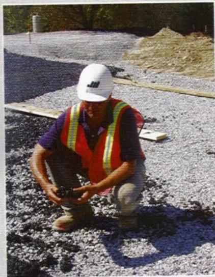
Site Superintendent Harold Lafoe checks the consistency of the porous asphalt.
